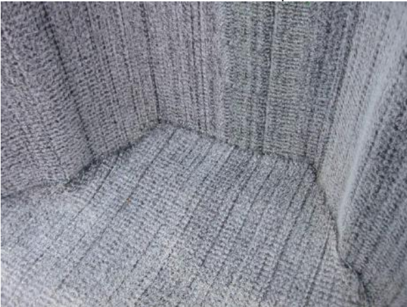
Beneath slab ActiTex cut to fit steel profile
