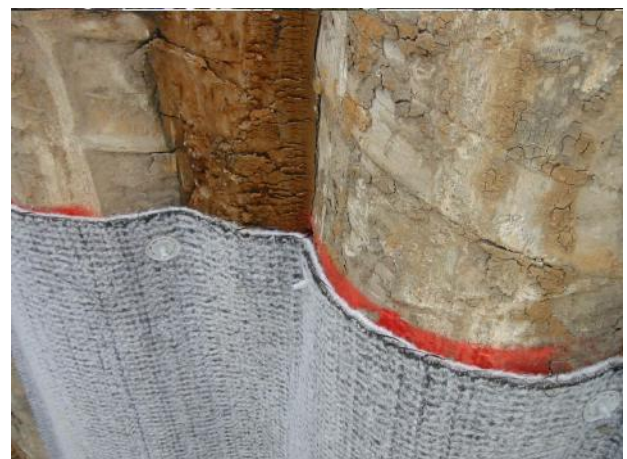
Securing ActiTex to contiguous pile (one third of pile face)
