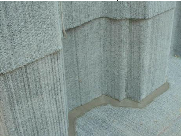
40mm Fillet of ActiTex paste (Granules & water)
