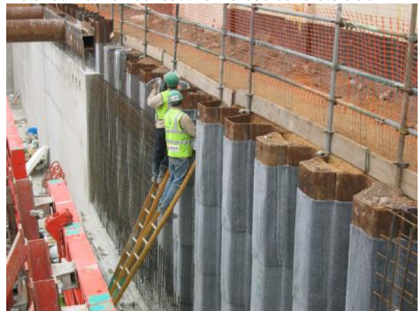
ActiTex continued up steel sheet wall
