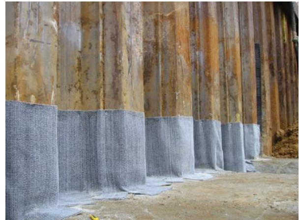
ActiTex splayed at wall/slab junction following contours.
