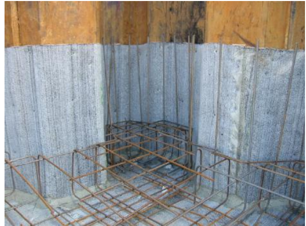
Installed Slab/wall ActiTex
