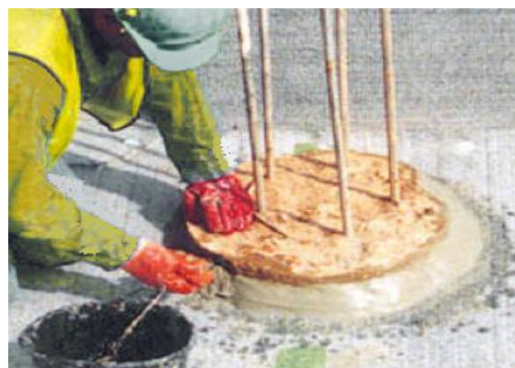
Application of 40mm Fillet of ActiFill paste to pile head
