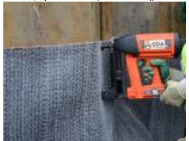
Fastened using washer head fixings
